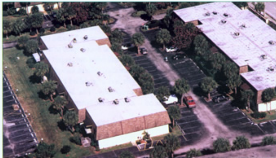
Building "D" shown left features a modified bitumen roof system.
